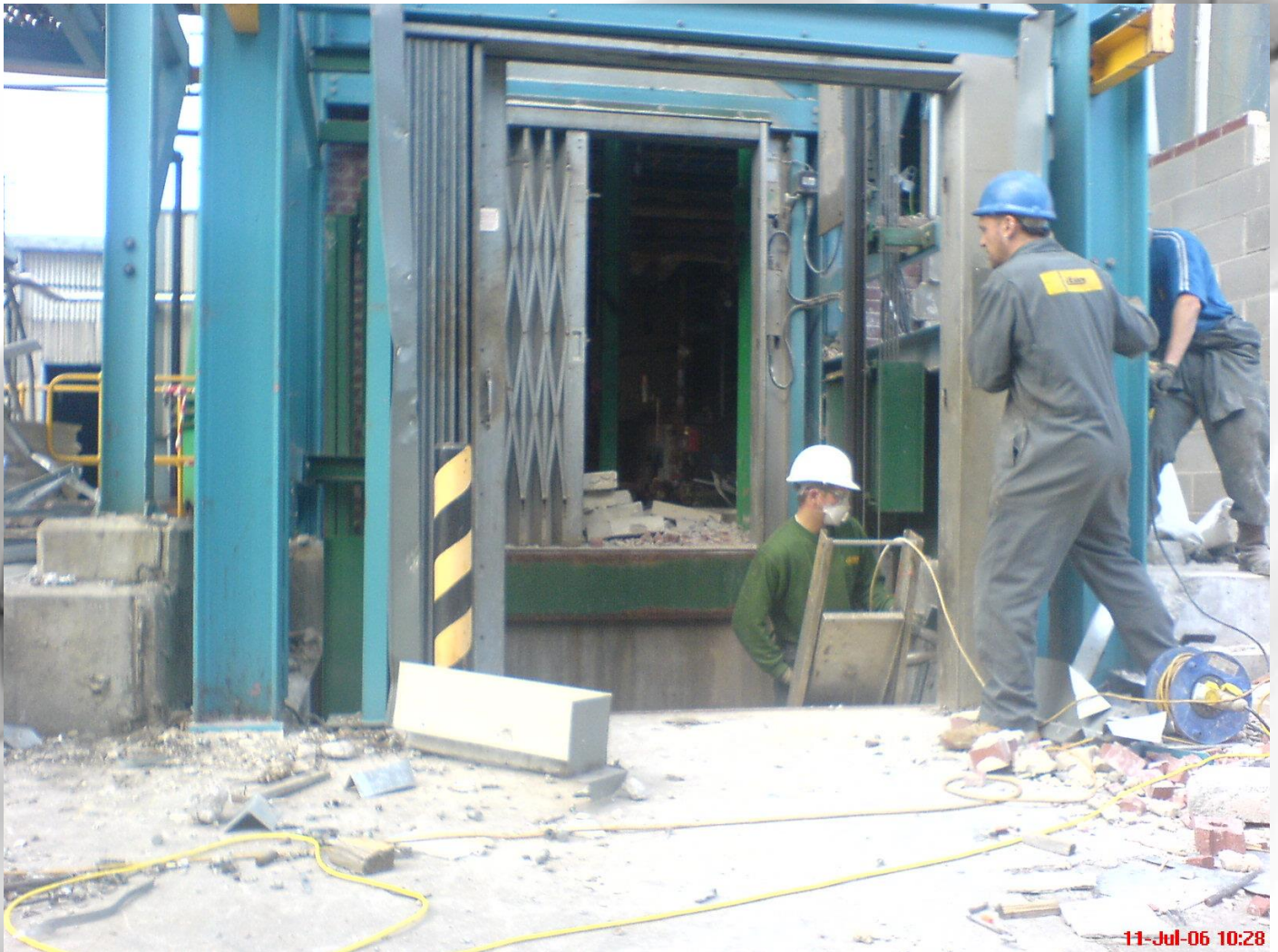
Above – Preparing the entry and exit points so the lift was free for removal.
